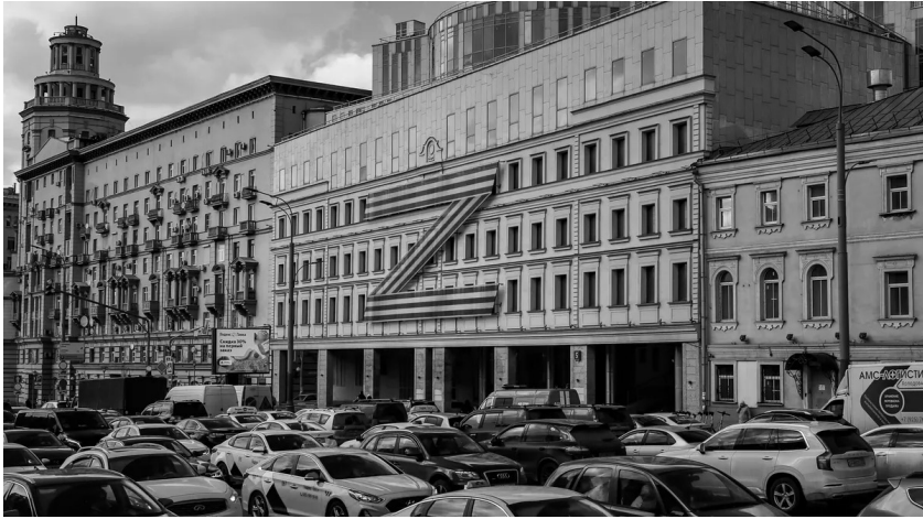
Above: Letter “Z” placed on the facade of the Oleg Tabakov Moscow Theater building in support of the “Special Military Operation”
